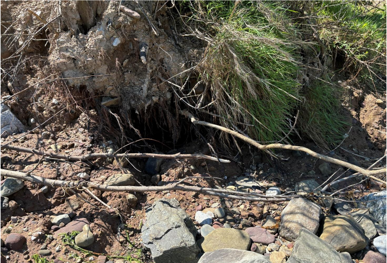
Figure 23 View of cliff toe notching between cross-sections F and G
