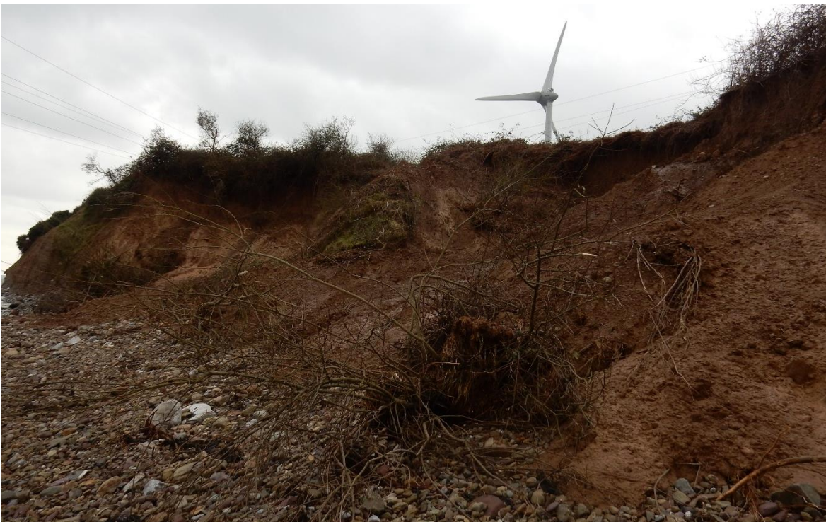
Figure 15 Area of collapse showing flatter slope
